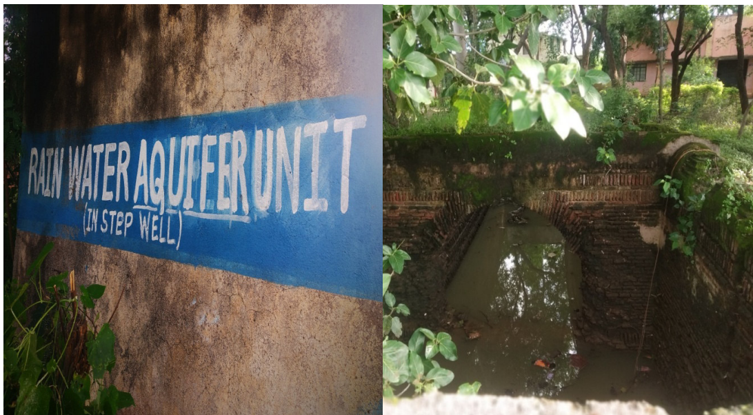
Open Space Rain Water Harvesting & Water Recharge System
